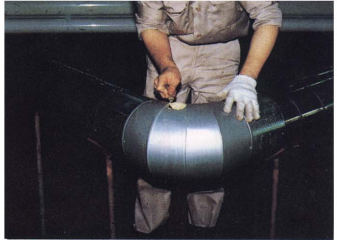
10. Trim excess foam.
