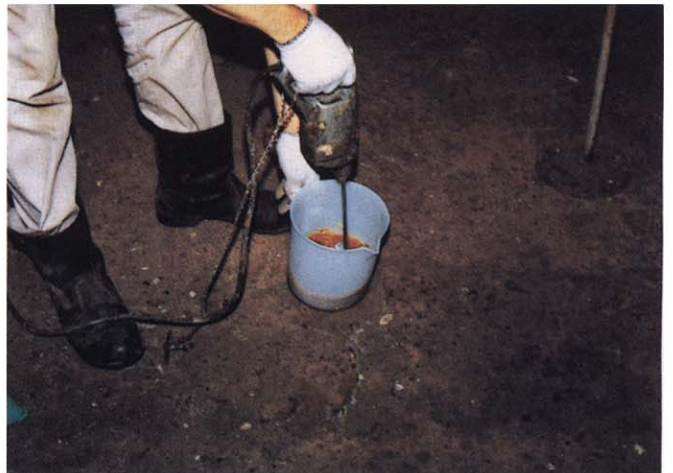
8. Pour Part B into mixing container first, then add part A. Stir and mix thoroughly for 25 to 30 seconds, preferably with electric drill and agitator attachment.
