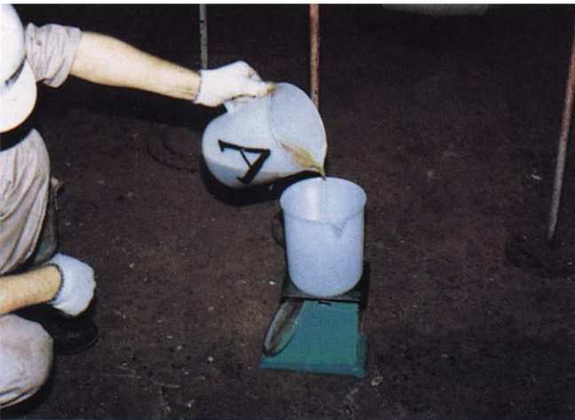
7. Pour required amount of part A (isocyanate) into measuring beaker. Pour required amount of part B (resin) into measuring cup.
